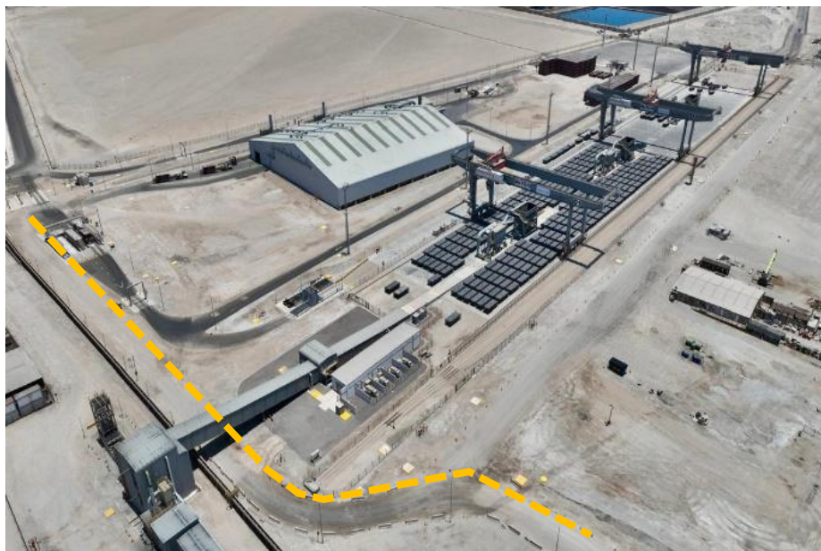
Vehicular route from the main access to the administrative building
